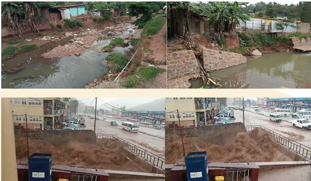
Figure 5: Illustration of flooding impacts in the sub-catchment (Source: RWB,2022)
