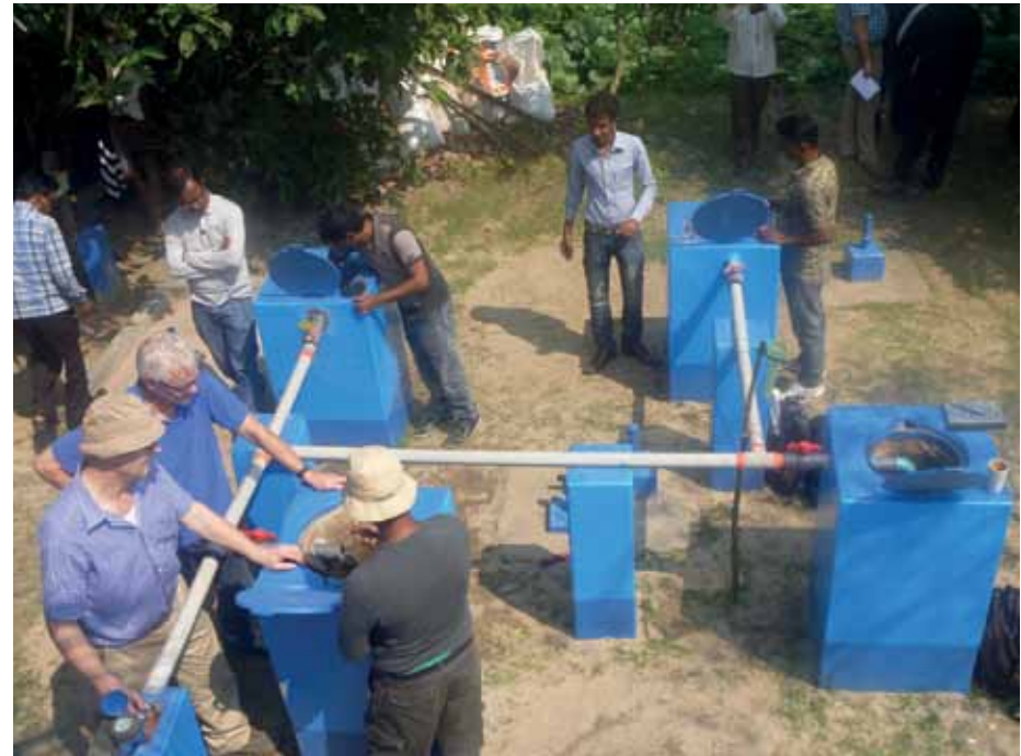
Photo 13. Field visit at a MAR pilot scheme.
