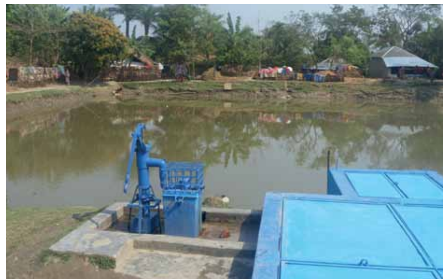
Photo 10. Underground MAR system in front of the pond.
