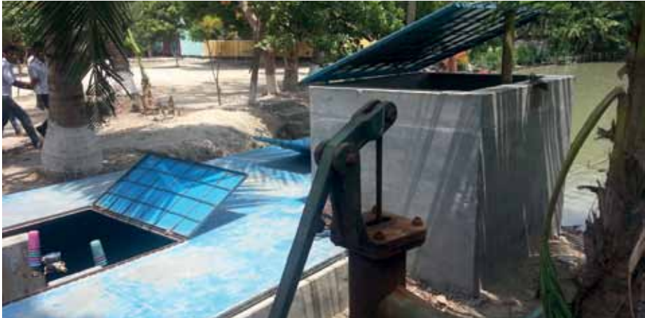
Photo 8. Underground MAR system.
