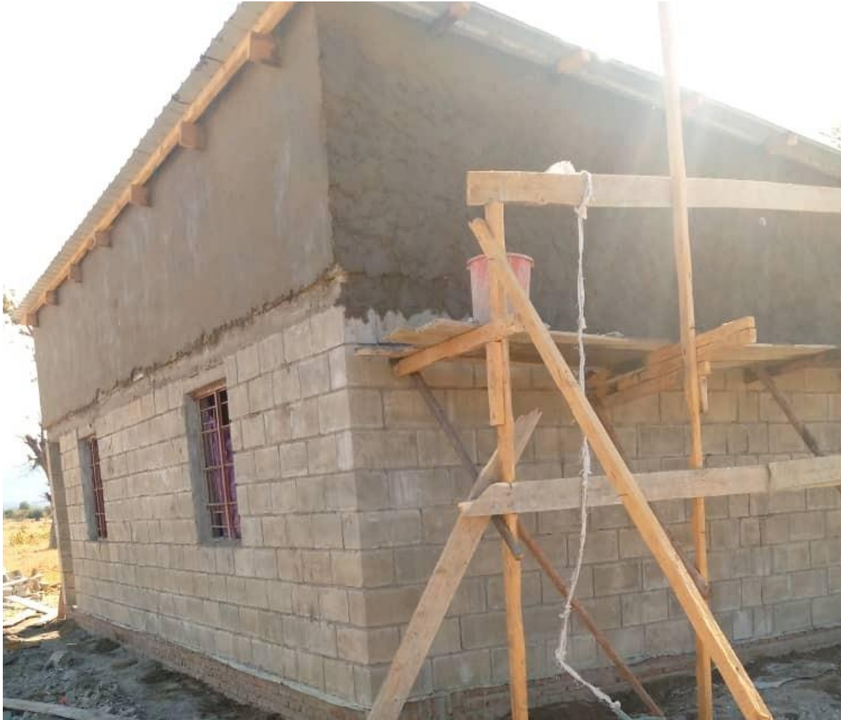
Figure 3. Pump house near completion at Kamuyisa WEF Demonstration site in Dedza
