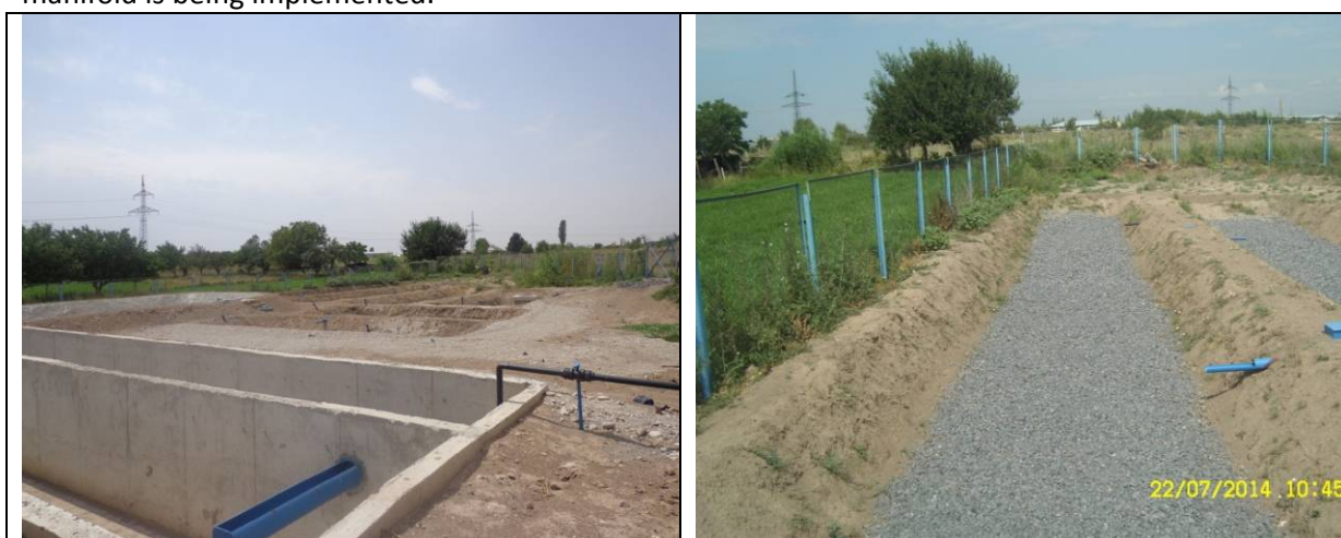
Reconstructed sedimentation pond
