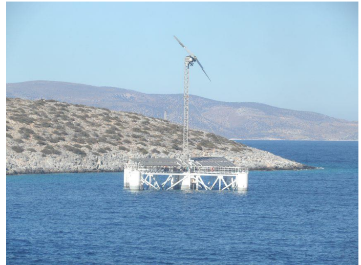
Irakleia Island, GR: patented floating desalination unit with WT
