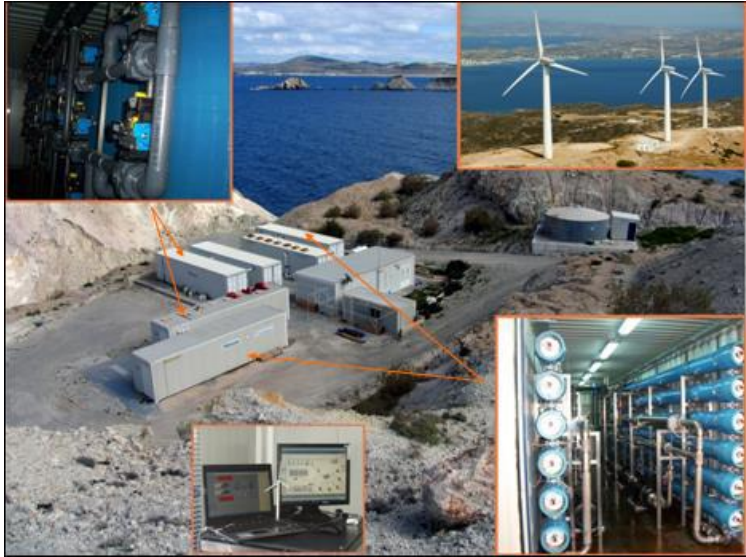
Pantelleria Island, IT: Hybrid desalination
