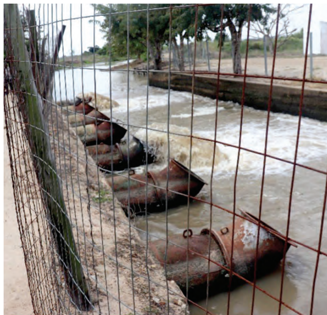
Abstraction of water for irrigation along the Pungwe River in Mozambique, intercepting the flow of water
