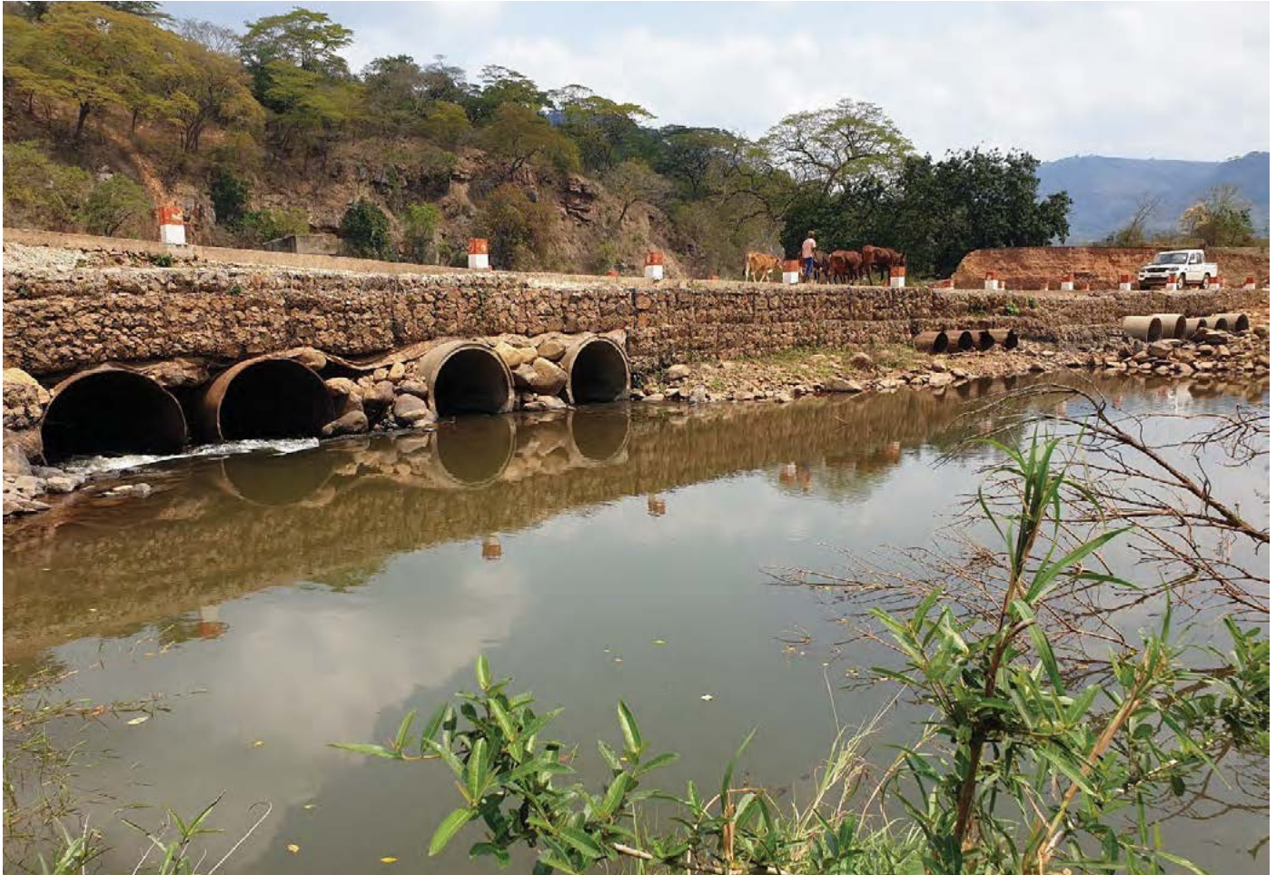
A bridge at Mucuiane, Mussorize River along the Buzi Basin in Mozambique. Photo Credit: GEF-BUPUSA Project
