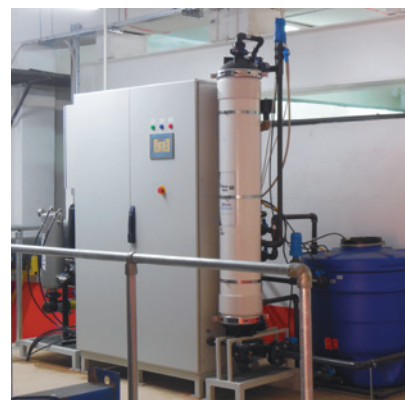
Fig.11: Above: Scheme of greywater recycling system with MBR technology (source: Catalogue of Technologies for Integrated Urban Water Management, 2014) Left: Greywater recycling plant with MBR technology, in Malta (source: SYSTEMA AZUD, S.A.)
