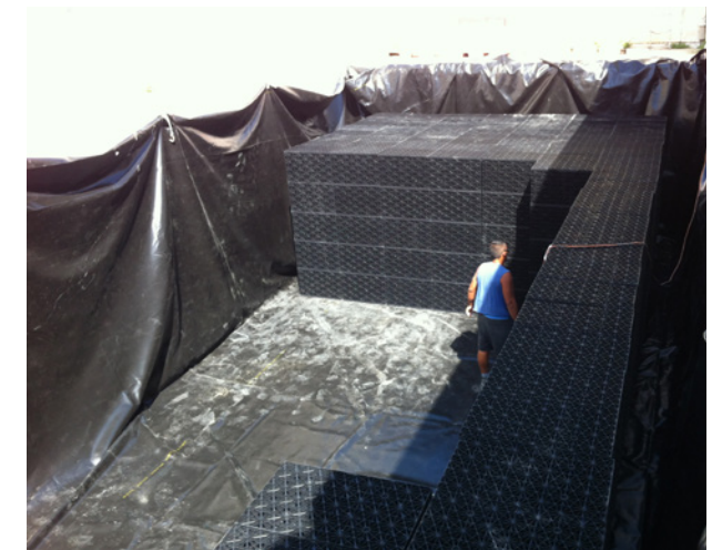
Fig. 8: Installation of a modular tank in Gozo, Malta (source: GWP-Med)
