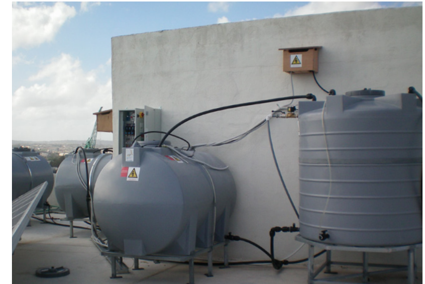
Fig. 10: Above: Chemical greywater recycling system installed in Malta (source: GWP-Med) Left: Chemical greywater recycling system installed in Cyprus (source: GWP-Med)
