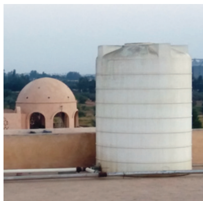
Fig.3: Above: Plastic rainwater harvesting tank installed by UNICEF-Rwanda. (source: E. Dusingizumuremyi, SuSanA Secretariat) Left: Plastic rainwater harvesting tank installed in Anafora, Cairo (Source: Mariela Antonakopoulou)
