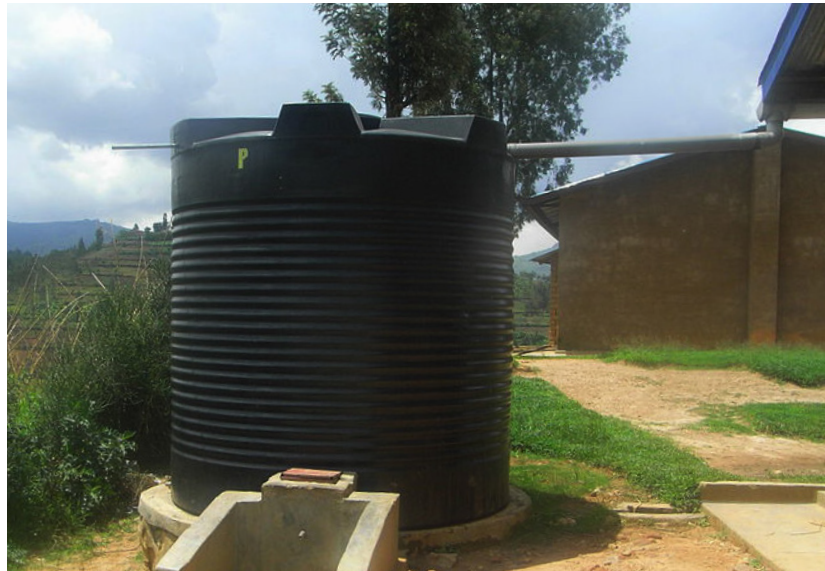
Fig.3: Above: Plastic rainwater harvesting tank installed by UNICEF-Rwanda. (source: E. Dusingizumuremyi, SuSanA Secretariat) Left: Plastic rainwater harvesting tank installed in Anafora, Cairo (Source: Mariela Antonakopoulou)
