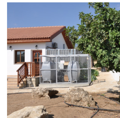
Fig. 10: Above: Chemical greywater recycling system installed in Malta (source: GWP-Med) Left: Chemical greywater recycling system installed in Cyprus (source: GWP-Med)
