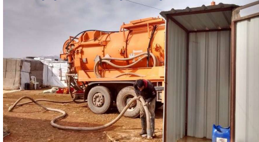
Desludging Truck Removing the Sludge from a Pit
