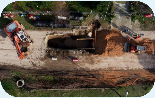
Installation of a rainwater drainage pipeline
