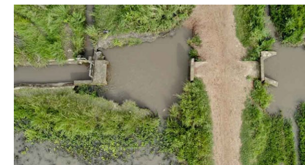
Aerial view of the Tulo Kongwa irrigation system, Tanzania. The system is unlined, a sign of inefficiency.
