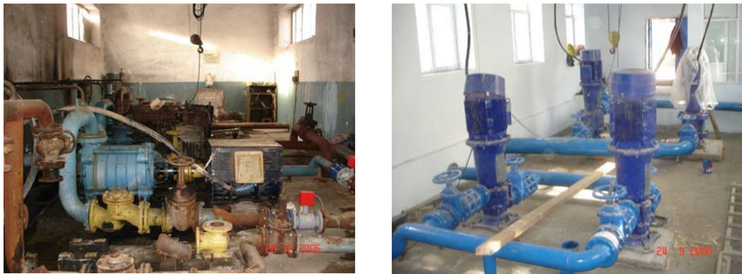
Picture 6.1. Aparan Pump Station in Armenia – prior and after reconstruction
