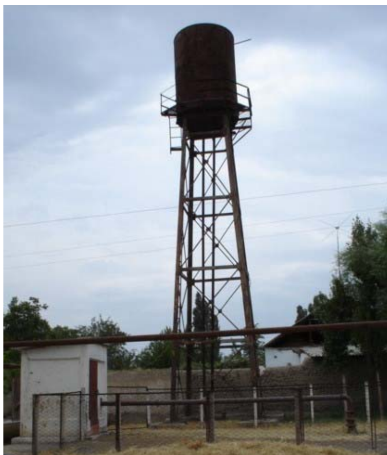
Picture 2.1. Water-tank tower in the rural area (Fergana Valley)
