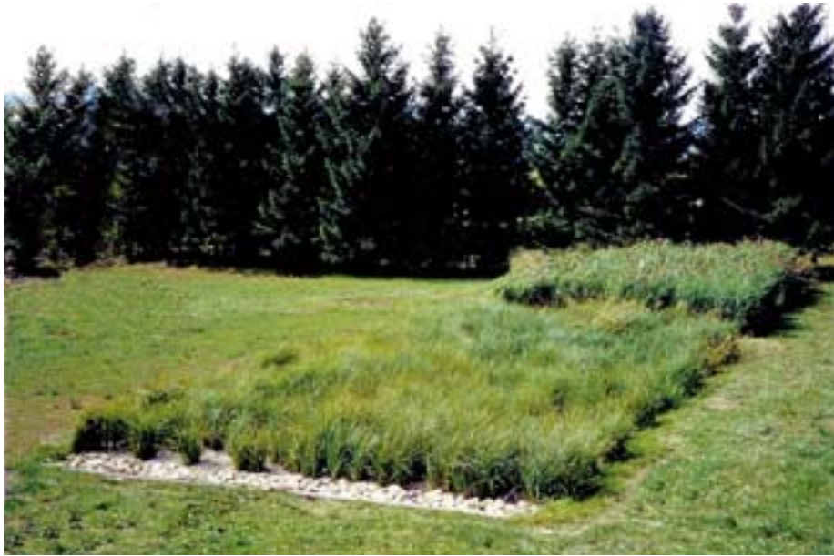
Constructed wetland in Gradisce, Slovenia
