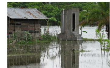
Figure 1: Urine Diversion Dehydration Toilets (UDDT) withstood the flood waters that resulted from a cyclone that struck southern Bangladesh in 2009 (source: A. Diepliere). More photos from this project: www.flickr.com/photos/gizecosan/sets/72157626407064863/
