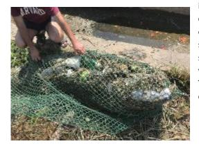
installed the waste collecting network on 805 breaking section of Artashat canal for testing purposes. The network was tested on the next day – August 3, after a 1-2 days' irrigation water shutdown and canal cleaning activities. Due to waste collecting system a considerable amount of agricultural and domestic waste was removed from the irrigation water.
