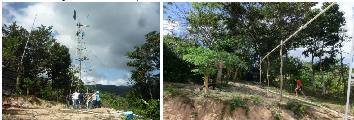
Image 4: Raising the tower Image 5: Irrigation conduction line
