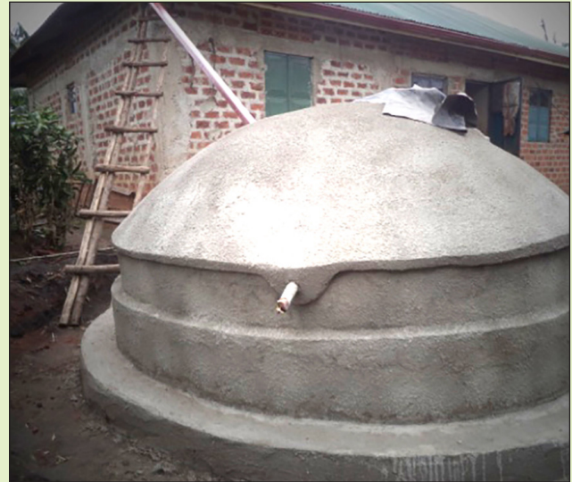
Completed underground water tank
