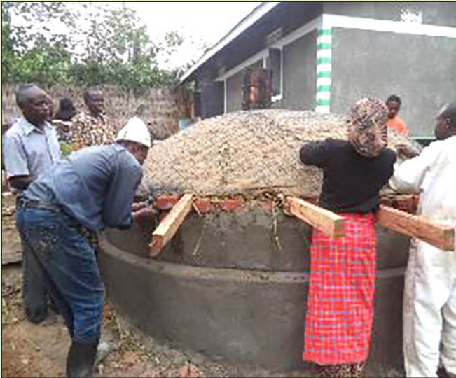
Community participation in construction of water tank
