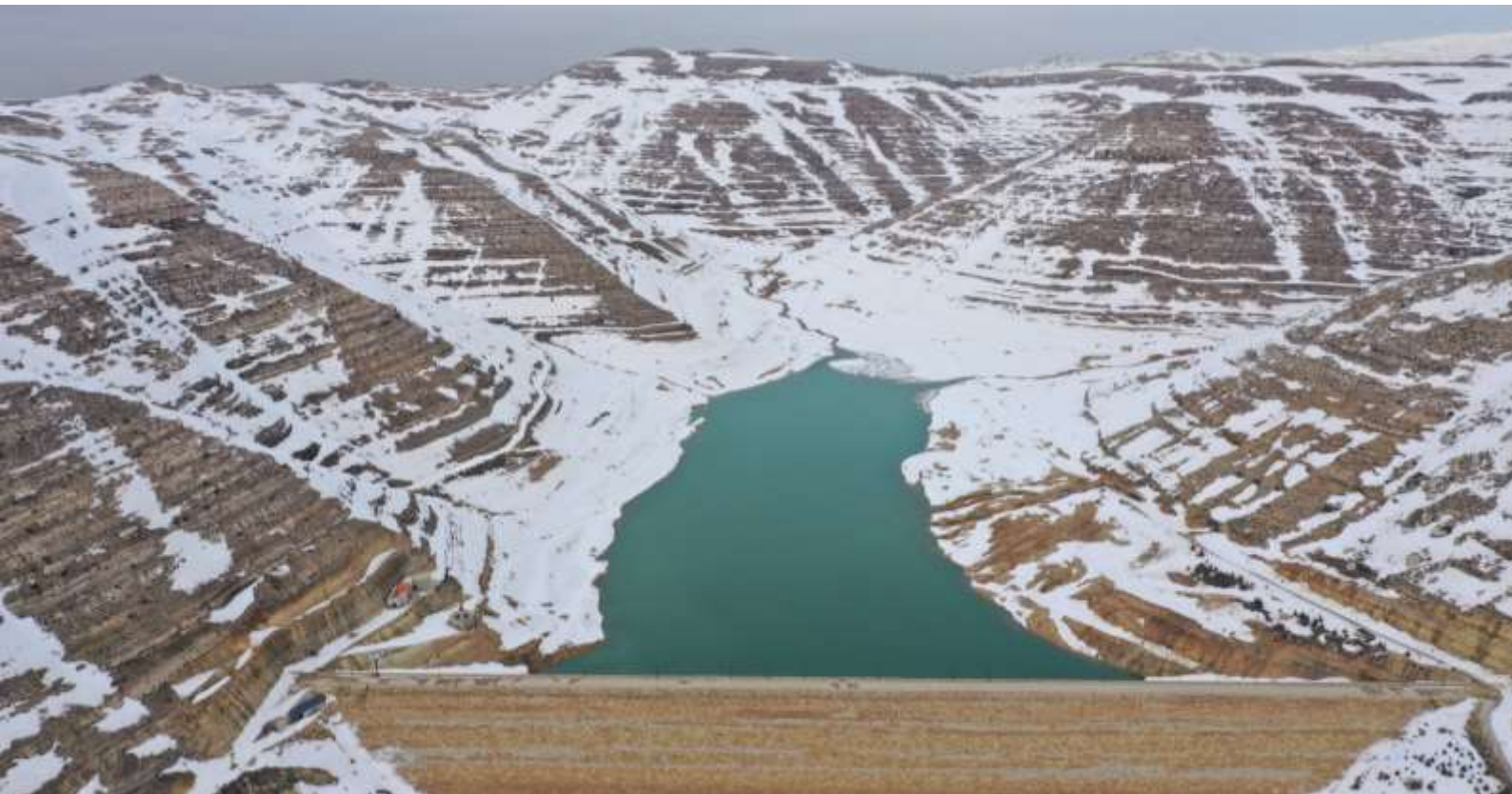
Chabrou dam, Lebanon © GWP-Med
