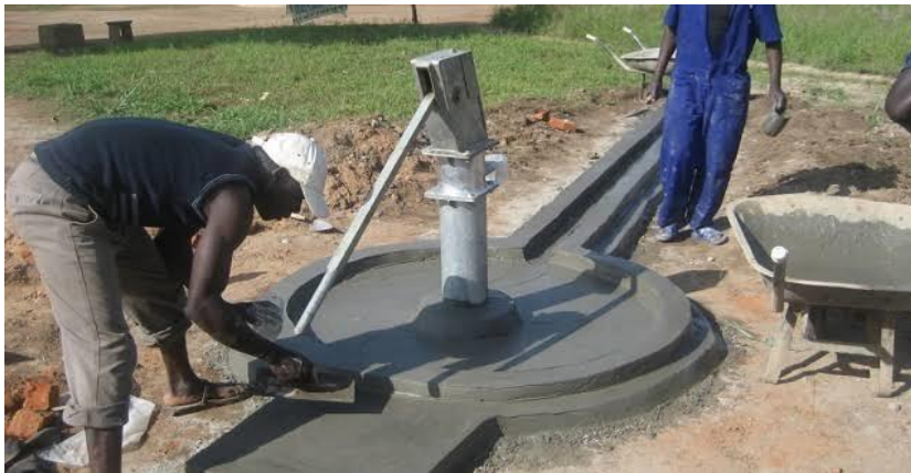
Fig 6: An improved borehole being constructed by some men volunteers in one of the villages.
