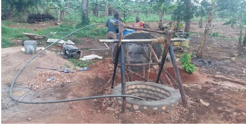
Fig 5: Improved shallow well being constructed in Nakanyonyi village
