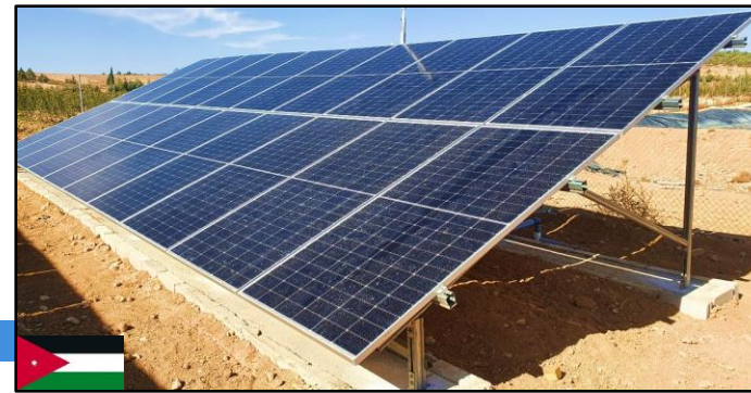
22 kWp on-grid solar PV system connected to a water drip irrigation system for Mr. Saleh Afash Al-Jazi's farm in Al-Achaari, Maan, Jordan.
