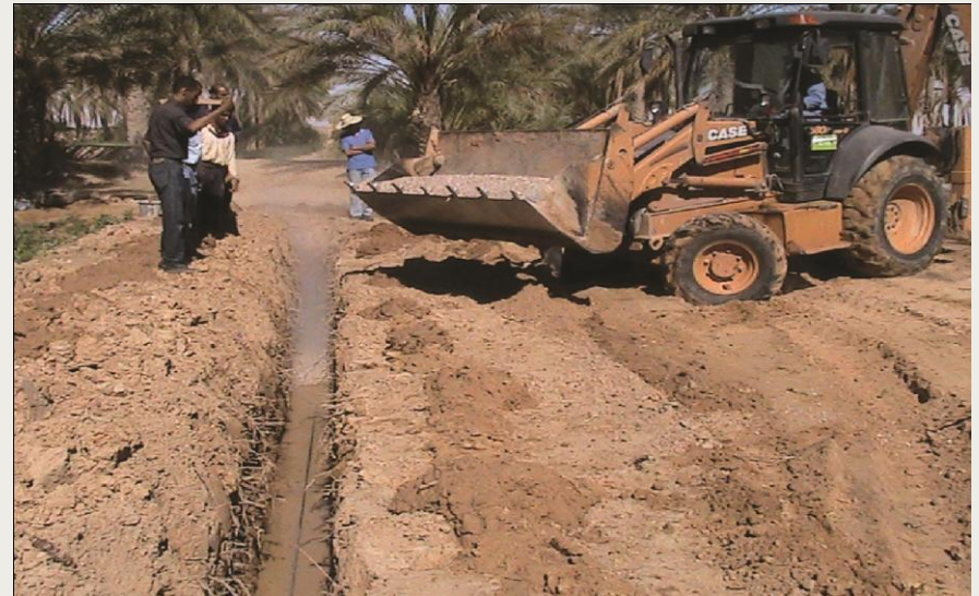
Drainage network construction
