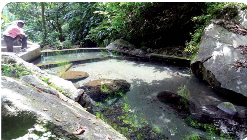
Sandy Bay water supply system
