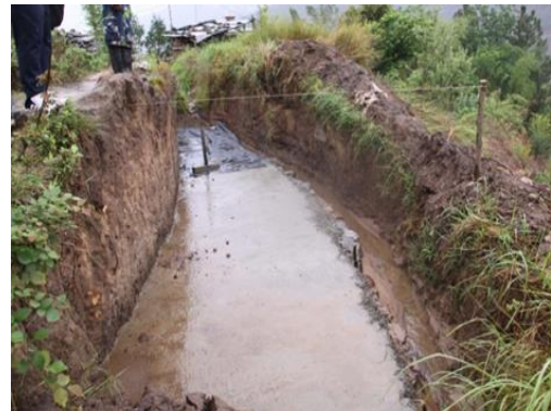
Foundation of outlet structure
