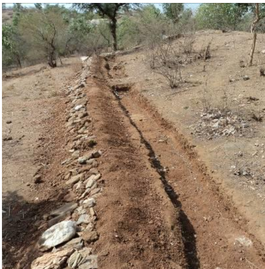
Construction of Continuous Contour Trench (CCT) – construction at Chuna Ka Wela village
