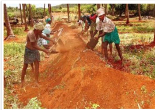
Farm Bund Work in Progress
