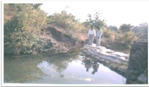
A Typical Vanrai Bund
