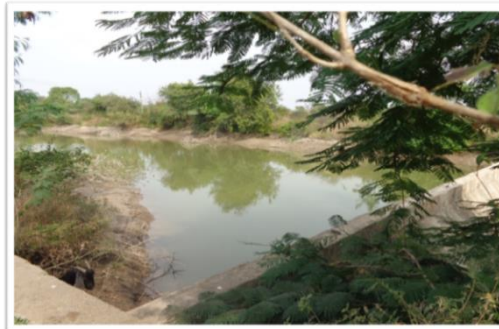
One of Kadwanchi's Cement Bunds
