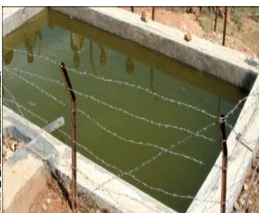
Water harvesting concrete pond
