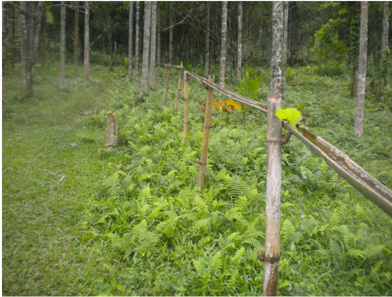
Supply of Drinking water from a spring to Sibbari (South Garo Hills) Primary School through Split Bamboo Pipes
