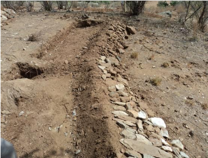
View of Gardonis at the time of construction (Kamalia village)
