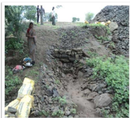
Stabilisation Pit for well recharging inlet pipe
