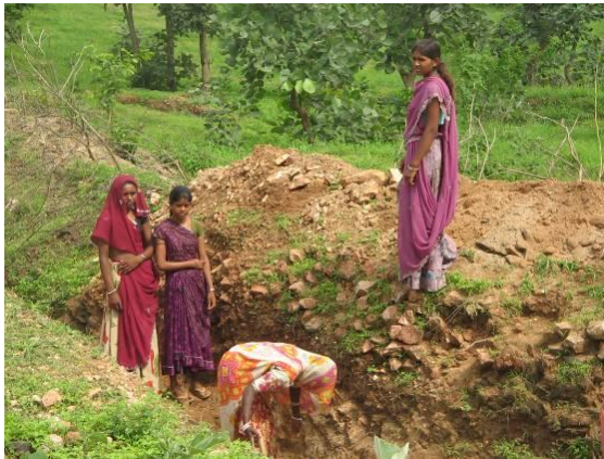
Construction of Cattle Protection Trench (CPT) in progress at Raila Village
