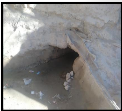
Destroyed Karez of Mastung
