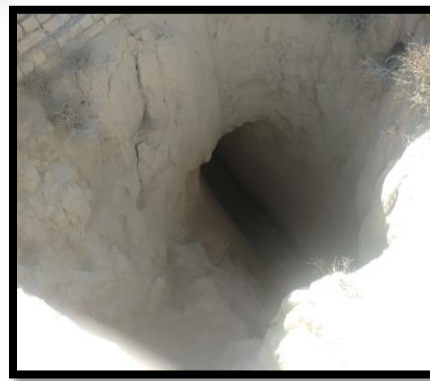
Rehabilitated Karez of Mastung
