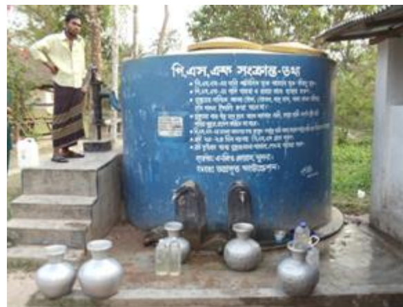
Hand Tube Well (left) and Pond Sand Filter (PSF) in the Polder area (right)
