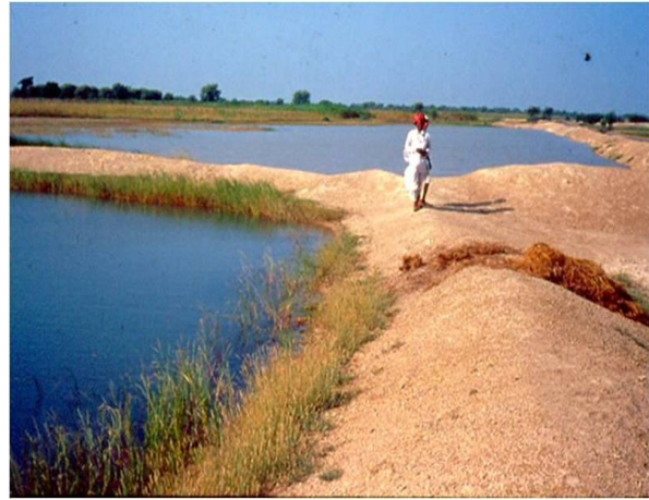
Water Harvesting Structures in series
