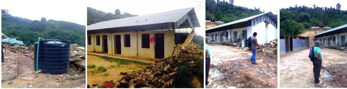
Damaged buildings were declared by government as unsafe. Mr. Batu, ECM of GWP Nepal observing the sites with a Technician from Smart Pani. Temporary structure built by school is visible.
