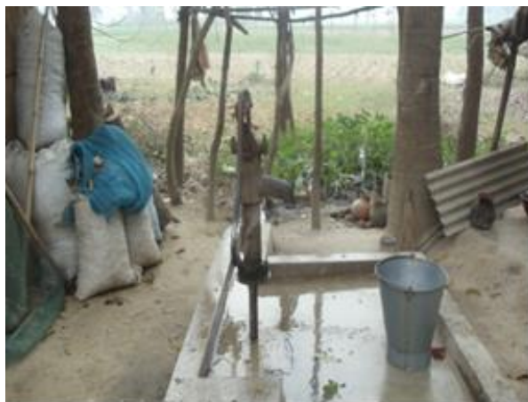
Hand Tube Well (left) and Pond Sand Filter (PSF) in the Polder area (right)
