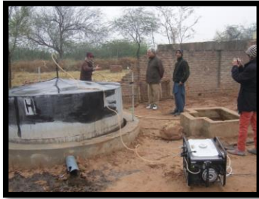
PWP Supervising the Biogas Water Pump
