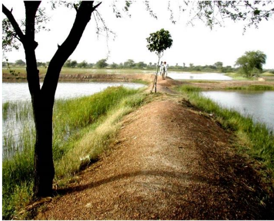
Water Harvesting Structures in series
