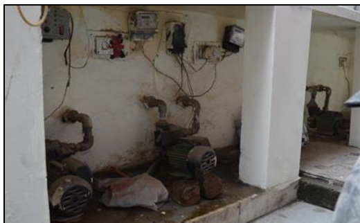
Three pumps being used for extracting ground water in a single house resulting in wastage of ground water and over use of energy
