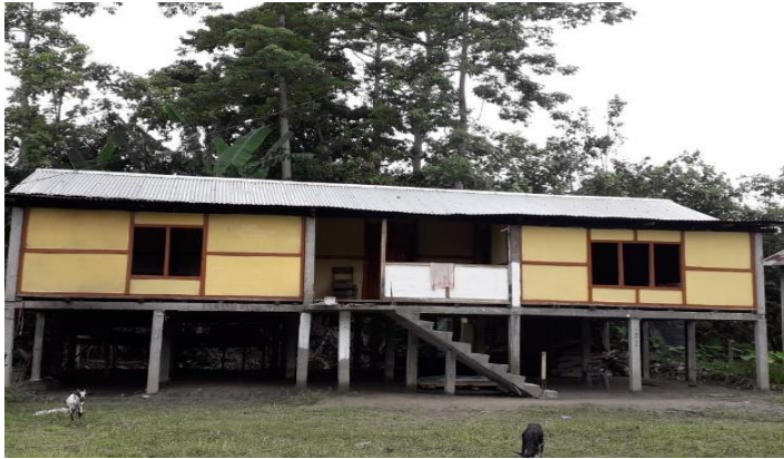
People live in stilted house to avoid flooding
