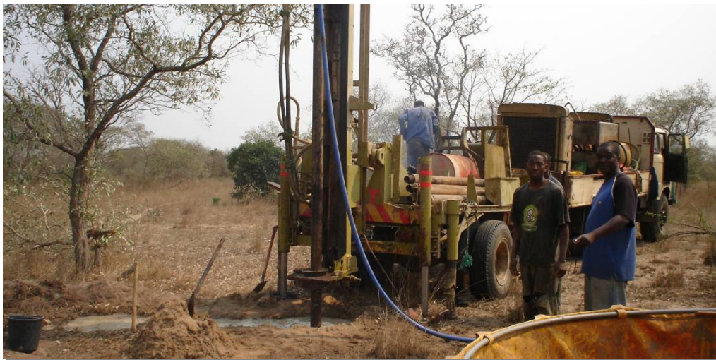
Drilling boreholes in Ndonga village, Mozambique
