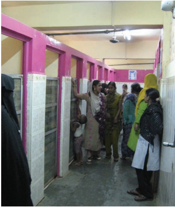
Figure 8.5: Community toilet blocks from the Slum sanitation Program (SSP) in Mumbai. The Mumbai SSP sanitation blocks provide the users with a sense of ownership towards the toilet block which helps to improve the operation and maintenance. © Stefanie Keller
