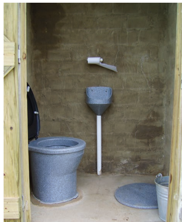
Figure 8.6: The UDD toilets in eThekweni were installed because it made sense as low-maintenance alternative to VIPs. The image shows the inside of the standard UDDT model. © Duncan Mara
