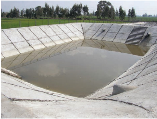
Figure 8.7: The decentralised treatment plant in El Moufty, Egypt today serves as a model for safer and more environmentally friendly wastewater treatment for smaller Egyptian settlements with populations between 3,000 to 5,000. © Duncan Mara
