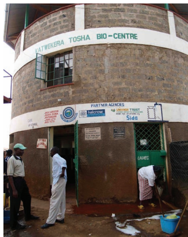
Figure 8.4: Communal bio-centres built in Gatwekera Village in Kibera are an example of how incremental improvements in improved sanitation services can provide an income source for community members, biogas for heating water and improved sanitation and hygiene. © David Crossweller
