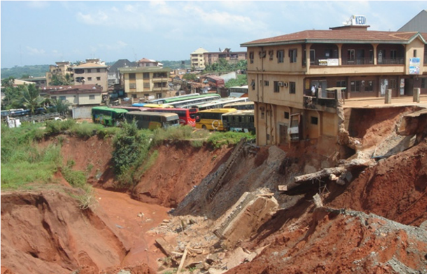
Figure 1.10 Buildings at Risk due to Gully Erosion, Omagba, Nigeria
