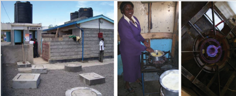
Figure B2.11.1 Lavatory and Wastewater Treatment Plant with Installed Biogas Generation Facility in Naivasha, Kenya
