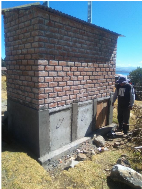
Sewage and urine treatment chambers
