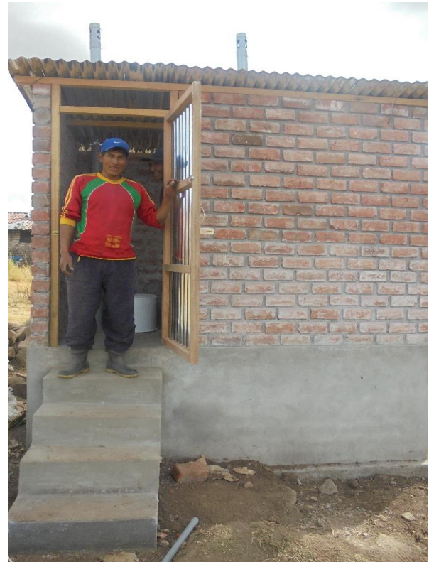
Built Ecological toilets in the Community
