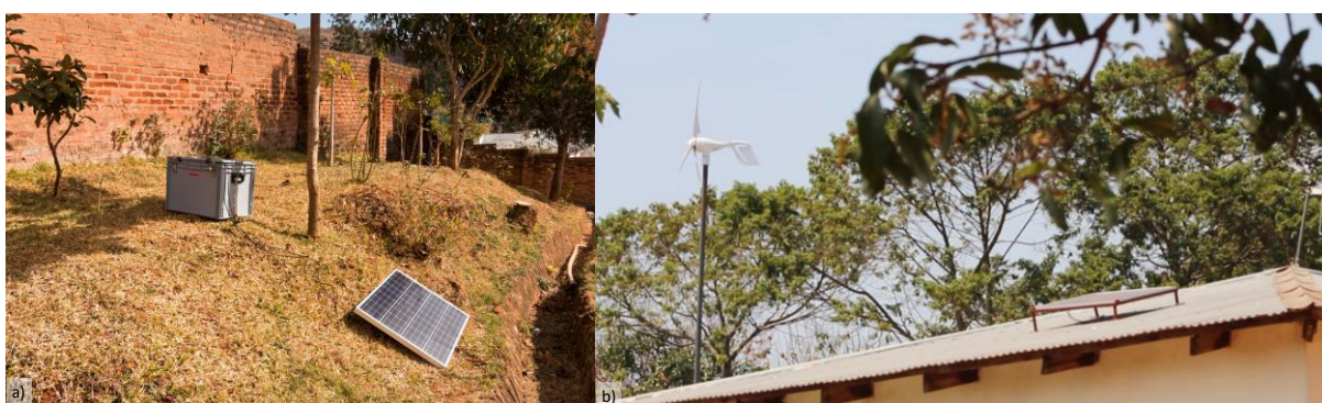
Figure 2: Recharge of batteries a) solar panel on the ground; b) solar panel and wind turbine installed on the roof of the Waste office building
