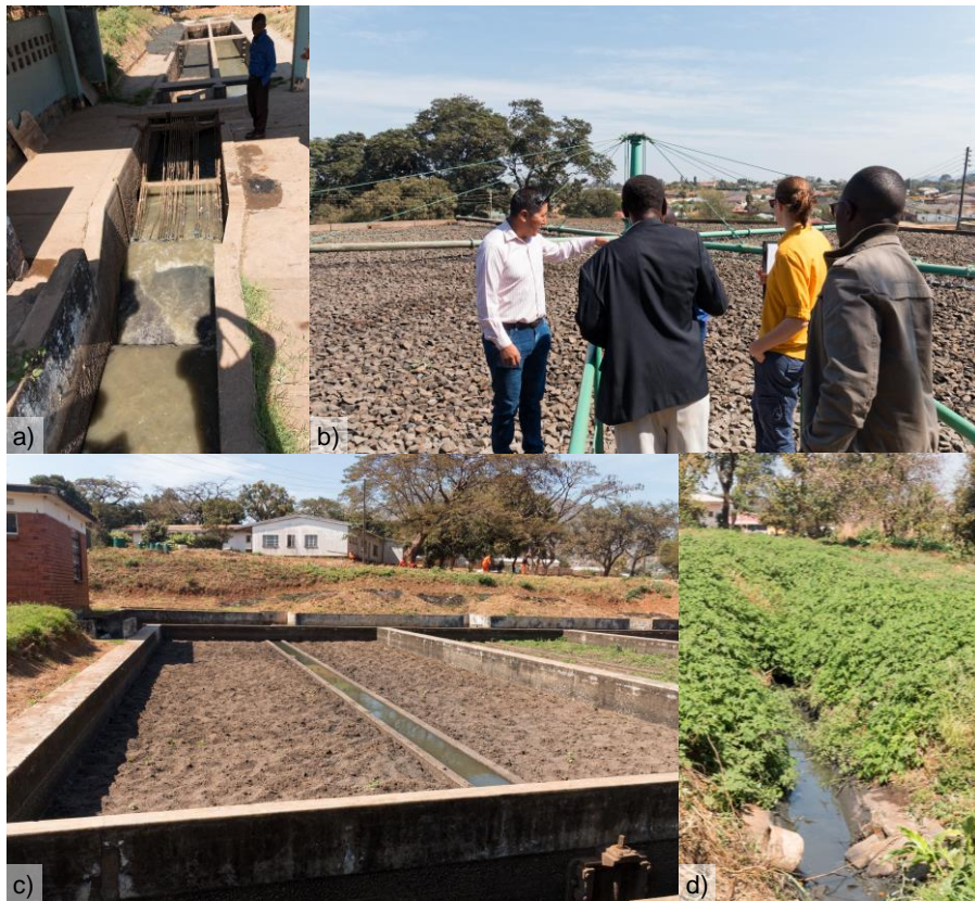
Figure 10: Impressions from Soche WWTP, a) Bar screen, b) Trickling filter, c) Effluent sand filter, d) Effluent stream (Pictures by Johannes Bousek)
