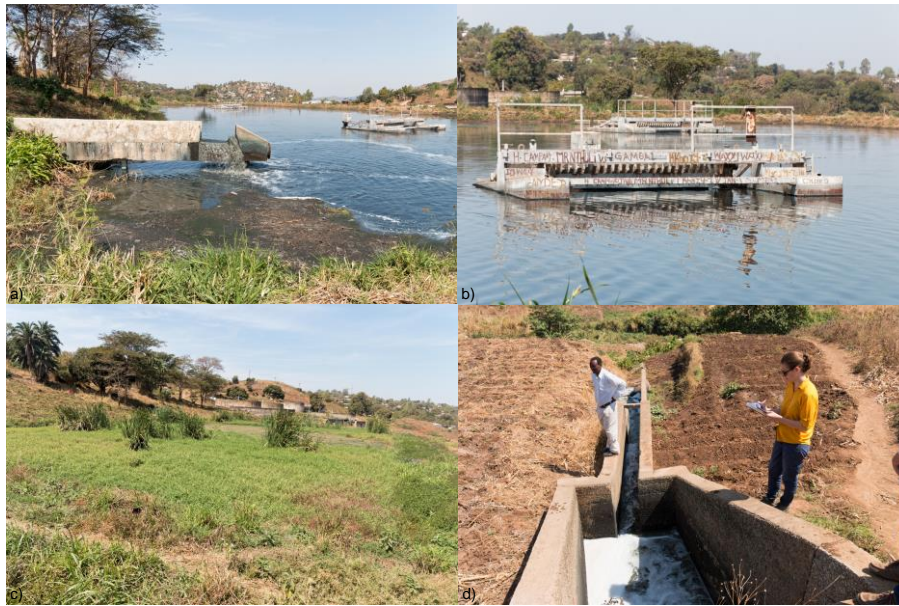
Figure 8: Impression from the Manase WWTP, a) Influent 1st lagoon, b) surface aerator (not operational), c) aerated lagoon, d) effluent structure (Pictures by Johannes Bousek)
