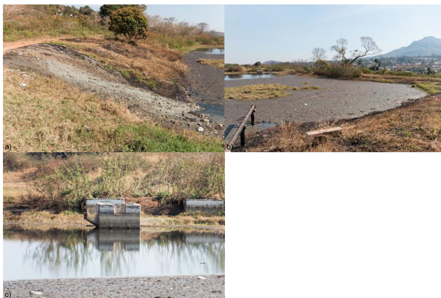
Figure 5: Limbe dumpsite a) dumping slope, b) view over the dumpsite, c) outflow structure (Pictures by Johannes Bousek)
