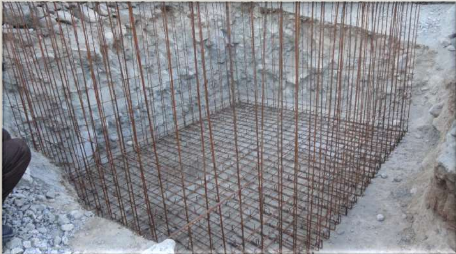
Re-bar of Storage Tank
