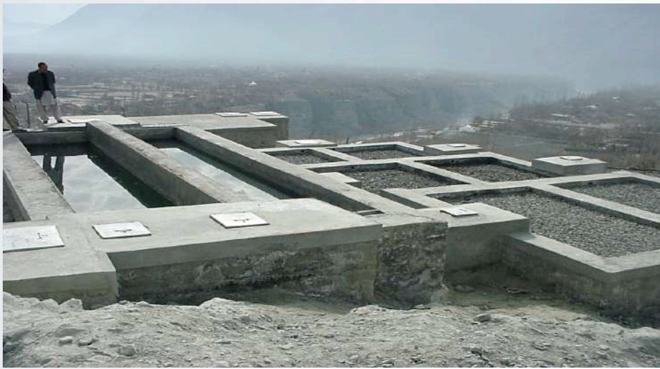
Up-flow Roughing Filter
