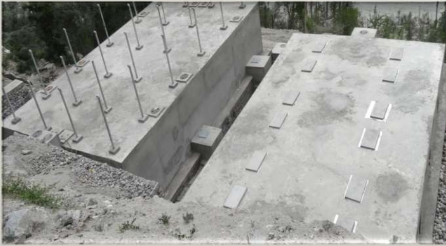
WWTP – Septic Tank + Bio-Filter
