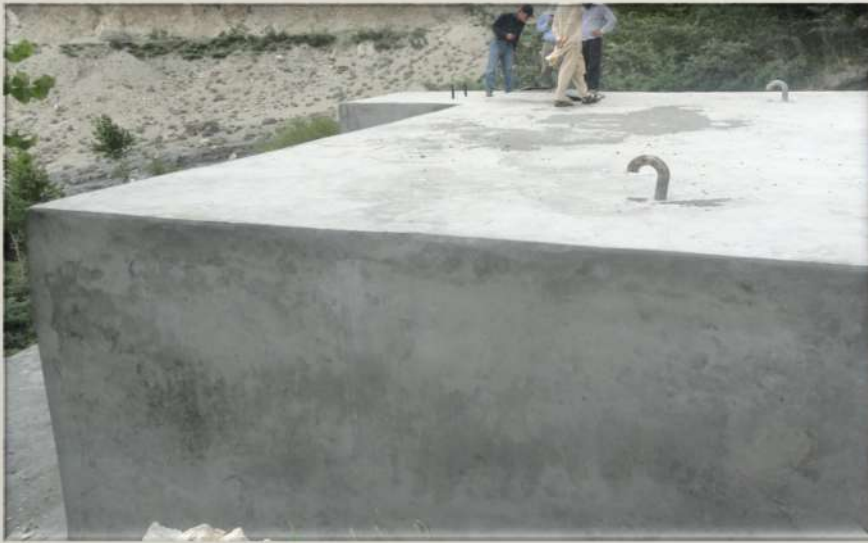
Water Storage Tank
