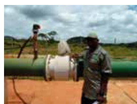
New protocols for monitoring water use and abstraction will drive efficiency & compliance
