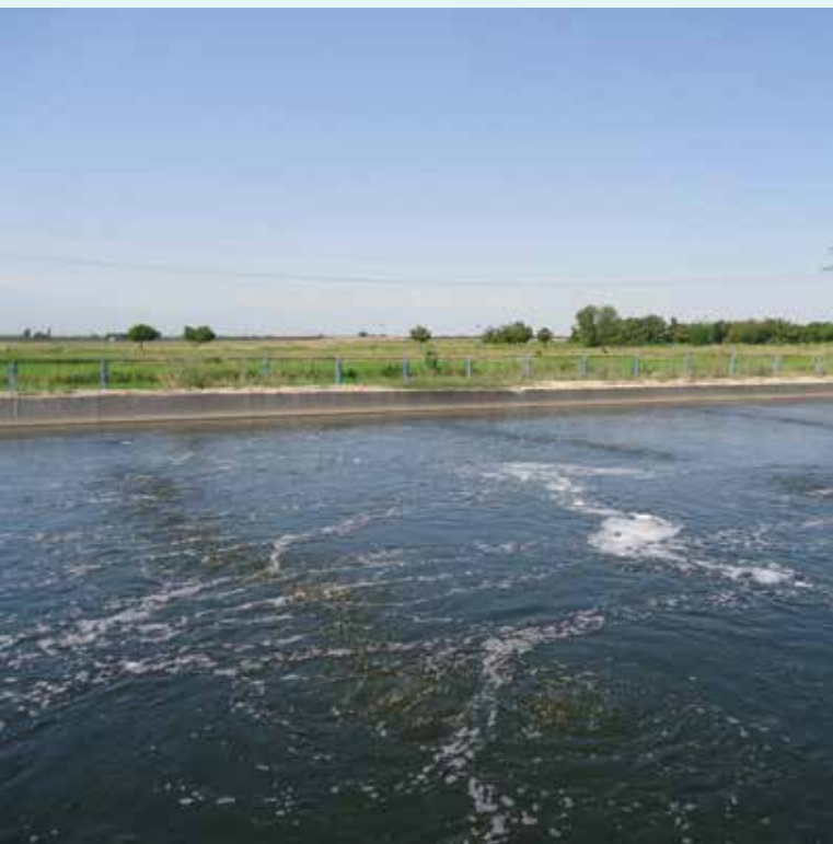
Improved wastewater treatment in Parakar, Armenia Credit: GWP Armenia
