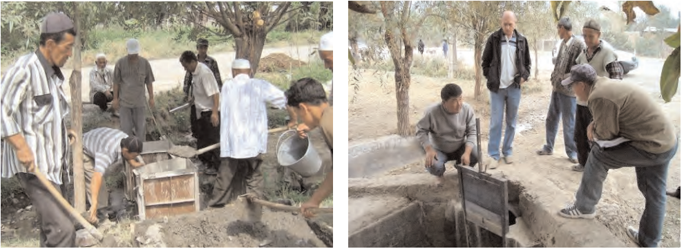
Figure 15. Construction of water metering devices at the WUA level, Kyrgyzstan
